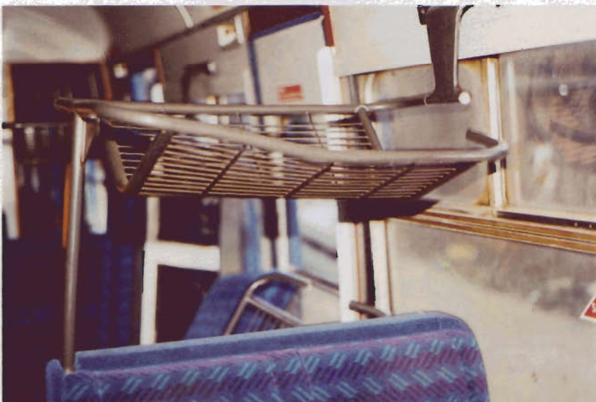
Fig 9. An interior view of a carriage of the Basingstoke train, showing damaged transverse luggage racks.
