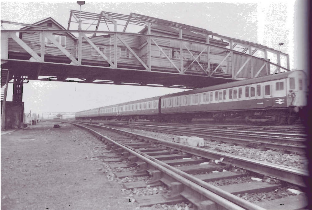
Fig 10. A view of Clapham Junction 'A' Signal Box with the relay room at the extreme right and the first third of the leading coach of the passing train.
