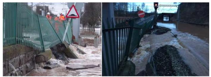
Figure 21 Wall along railway at entrance to Viaduct Estate that collapsed during the flood event
